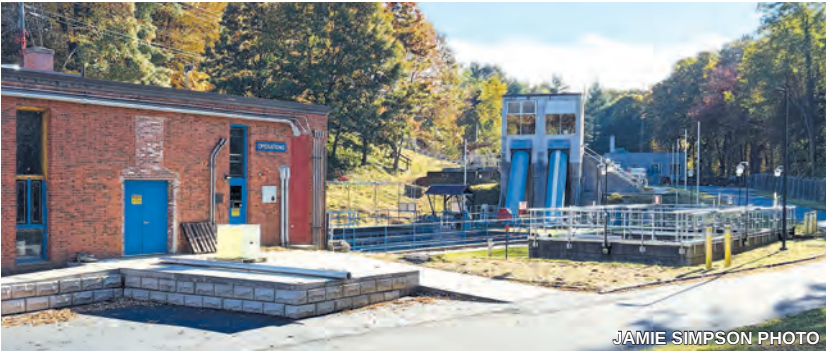
When one of Montague’s few remaining large employers closes next year, the town’s wastewater plant anticipates losing nearly a quarter million dollars of annual revenue in sewer fees — and a source of good, high-energy food for its microbes.
