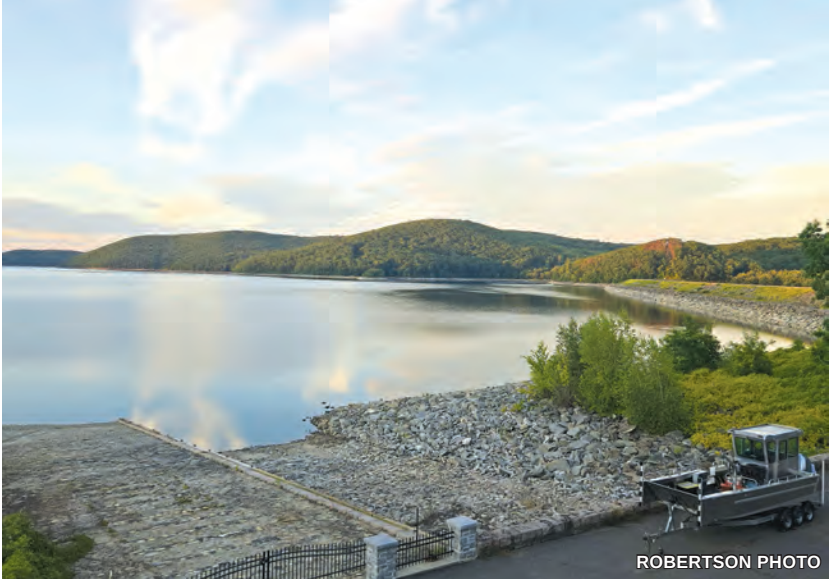
At the Windsor Dam in Belchertown, the Quabbin’s depleted state is visible.
