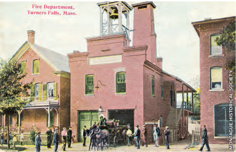
The Turners Falls Fire District built the fire station on Third Street in 1873.
