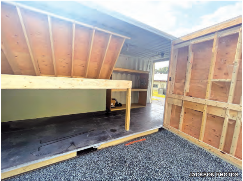
Inside the training lab: Nooks and crannies were carefully designed to simulate an attic crawlspace (at left) and, behind plexiglass, wall cavities of various shapes.
