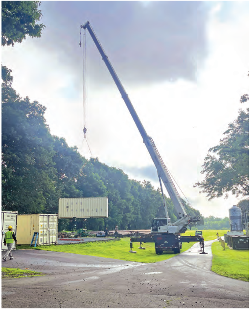
Carl Woodruff of Oxbow Design Build heads over to help the crew position the “attic” training lab on the pad.
