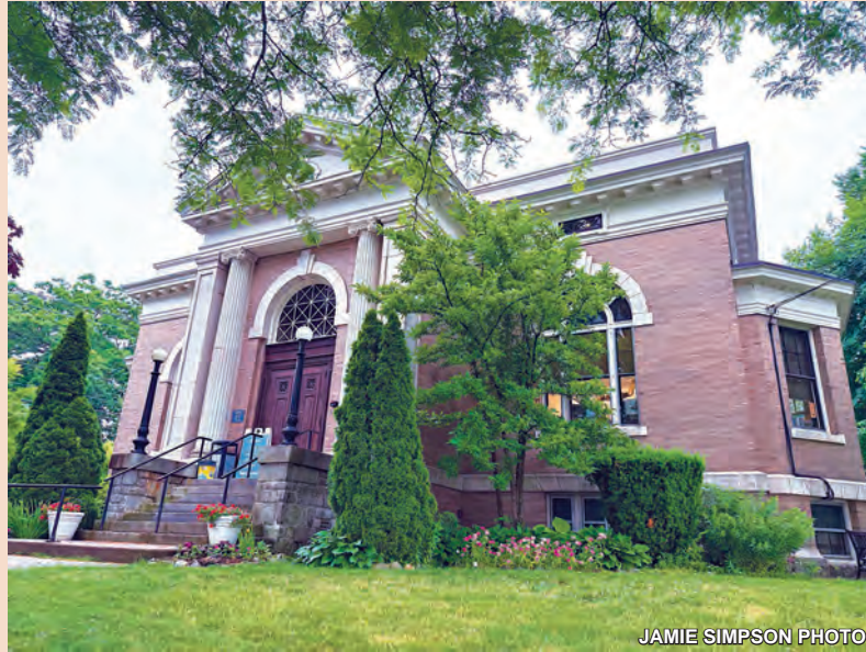
The Carnegie Library in downtown Turners Falls would be replaced by a new, larger building at 38 Avenue A if a majority of Montague voters approve a debt exclusion for the project next Wednesday, June 24.
