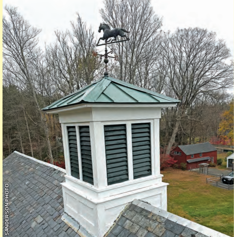
The cupolas on 19th-century barns were designed to vent heat and moisture.
