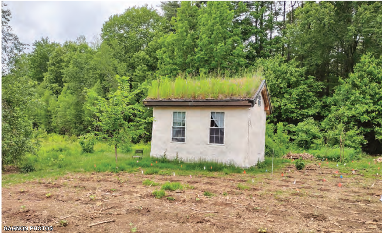
Big Foot’s strawbale studio, with its grass roof.
