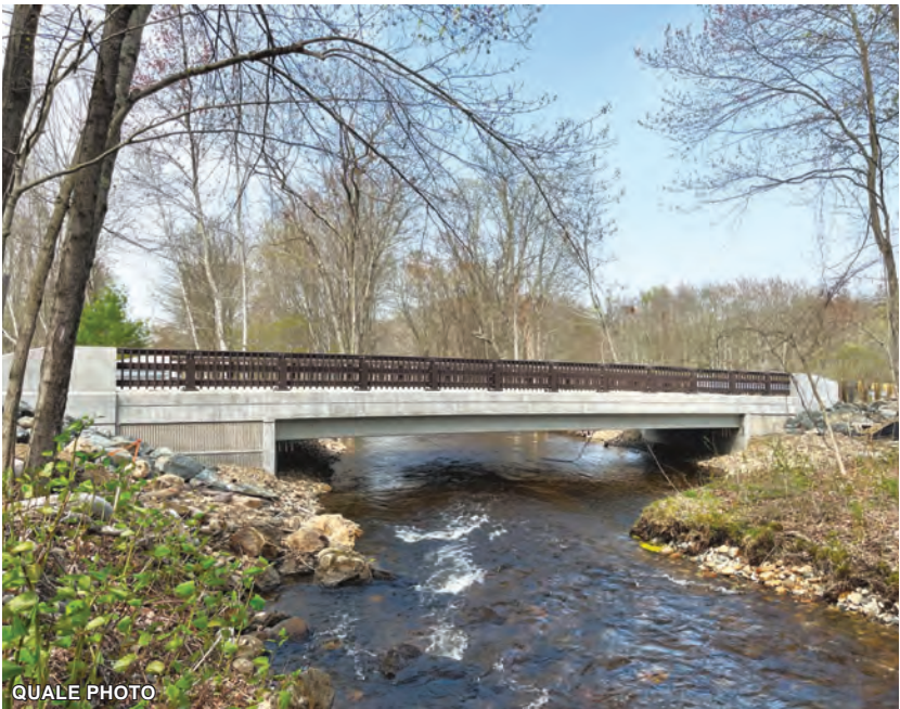
The bridge’s west abutment, seen above at left, was formerly set in the river itself, constricting its flow. The new, longer span allows it to rest on both banks.
