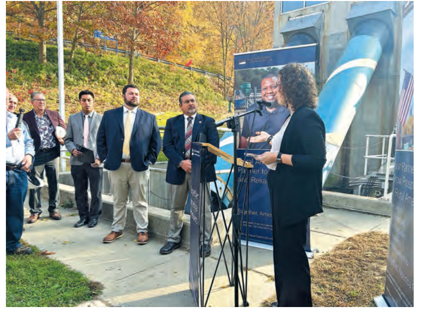
CWF superintendent Chelsey Little addresses the visiting dignitaries on Wednesday. The plant's iconic twin Internalift-brand Archimedes screw pumps, last replaced in 2002, lift the sewage from the plant's primary clarification tanks uphill to the secondary clarifiers. Little said that if both aging pumps were to fail, the plant and its surrounding wetlands would be flooded with sewage in a matter of hours.
