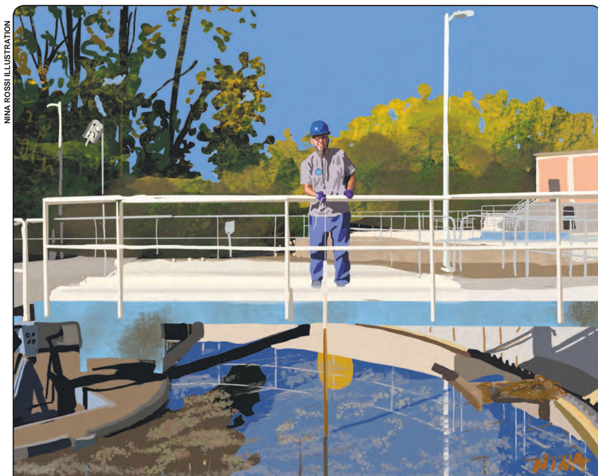
On a recent brilliant fall day Andy Skjiff, laborer-operator at the Montague Clean Water Facility, dips a tube into the secondary clarifier tank in order to measure the "solid stuff" at the bottom.
