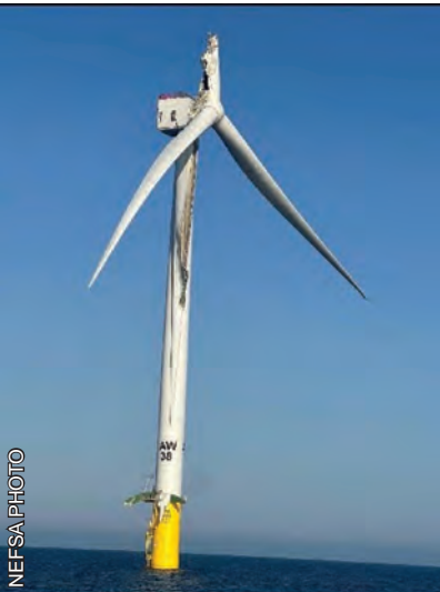
A 107-meter blade broke off the Vineyard Wind 1 turbine this summer. Photo courtesy of the New England Fisherman’s Stewardship Association.
