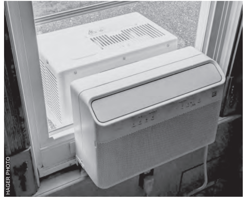
U-shaped air conditioners, such as this model by Midea, isolate the two ends of the cooling system from each other.
