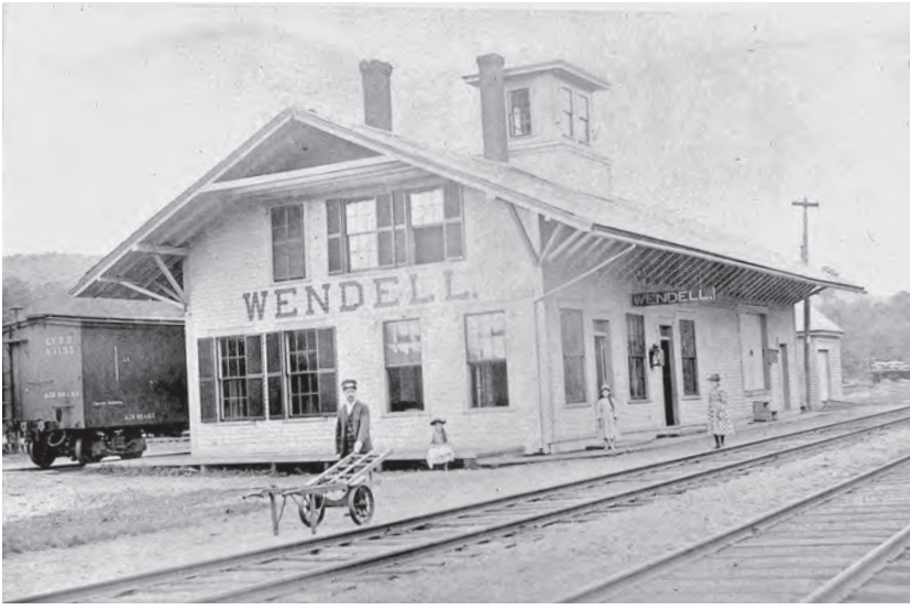
Wendell Depot Station, built in 1849 and demolished in 1942.
