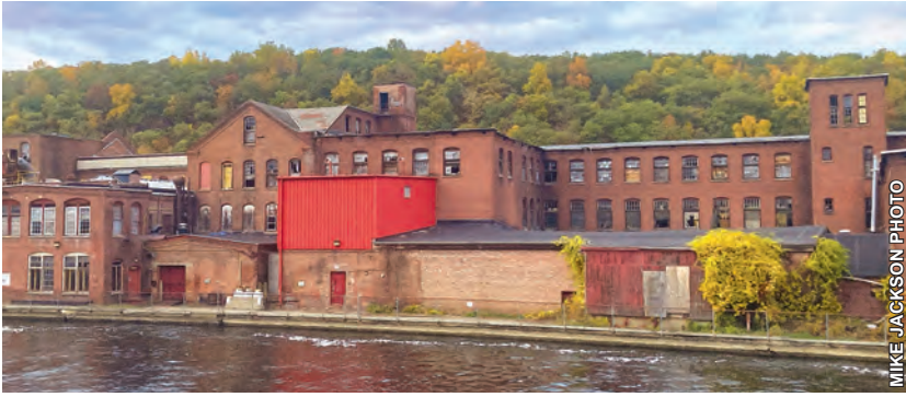
Asbestos in the Strathmore Mill's roofing may help the town secure funding for a partial demolition of the distressed complex.
