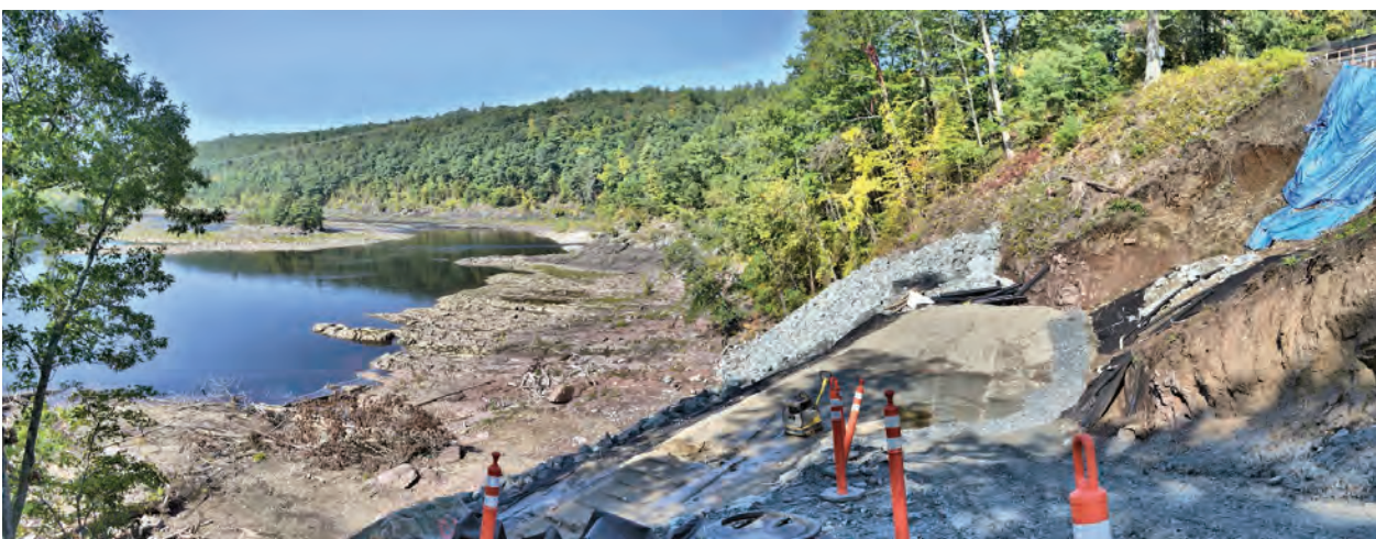
Ed Gregory took this photo of work being done to shore up the Connecticut River bank along Route 2 in Gill on October 1. “This image shows the very base of the landslide area being prepared for embankment reinforcement,” Ed writes. “Huge boulders will be laid in at the base of the wash, and later rock fill will be buttressed up against this wall of boulders to contain the steep slope.”
