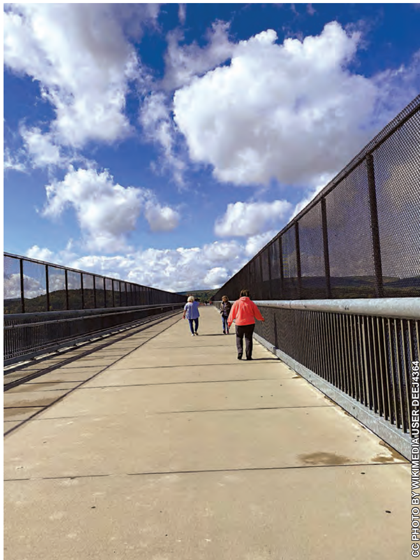
A railway bridge walkway over the Hudson in Poughkeepsie.
