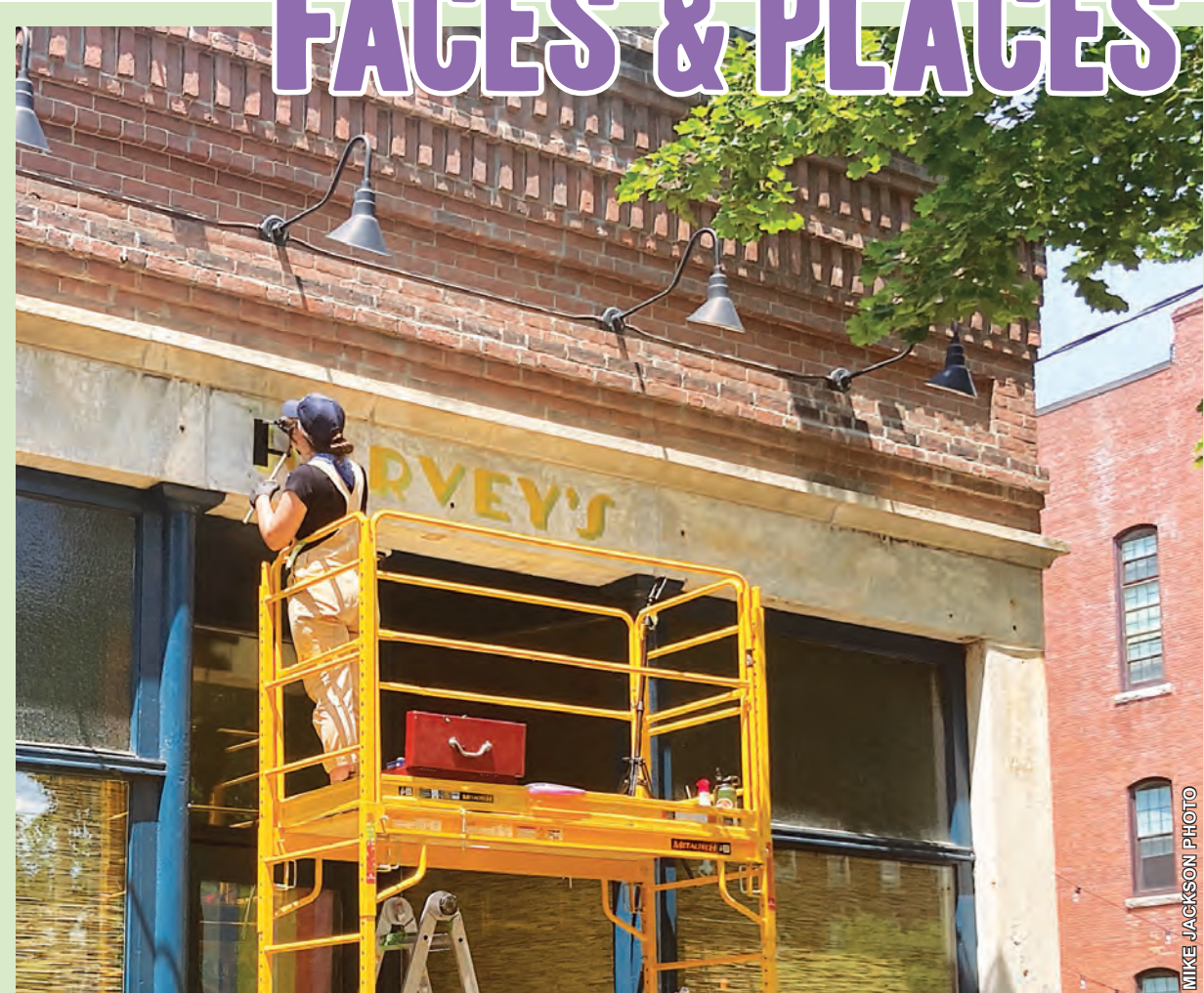
Wednesday afternoon found Turners Falls sign artist Jess Marsh painting crisp black letters straight onto Harvey's, soon to be the newest restaurant on Avenue A. A day earlier, Marsh had applied the drop shadow in gold leaf. Marsh worked slowly and methodically, as the marble lintel afforded no room for error. She told the Reporter that while she enjoys painting her signs directly onto buildings, she rarely gets a chance; at Harvey's, restaurateur Evelyn Wulfkuble co-owns the building and can make such bold decisions. Marsh's business, Hired Hand Signs, is headquartered on Third Street.
