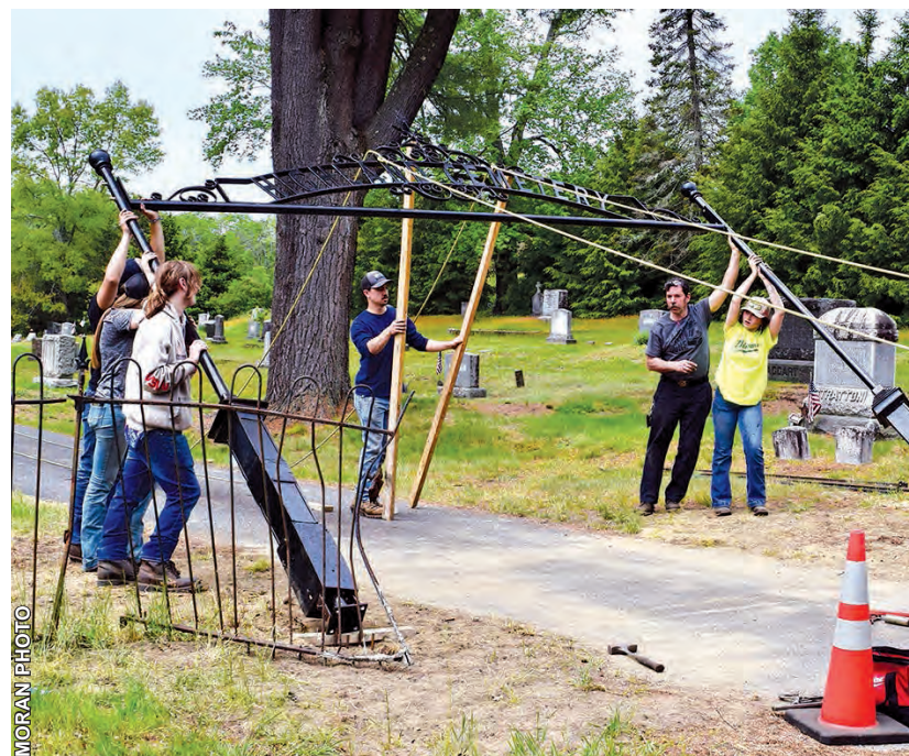
Students from Franklin County Technical School welding and metal fabrication program raise the newly wrought gate at Highland Cemetery.
