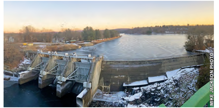
The hydroelectric relicensing process has dragged on for over a decade now.
