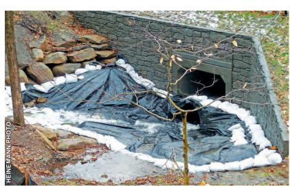
The botched culvert has been temporarily patched with sandbags and plastic sheets.
