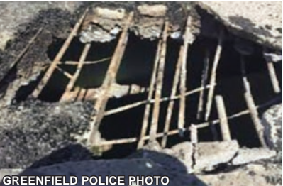
A 2015 hole in the bridge’s deck.
