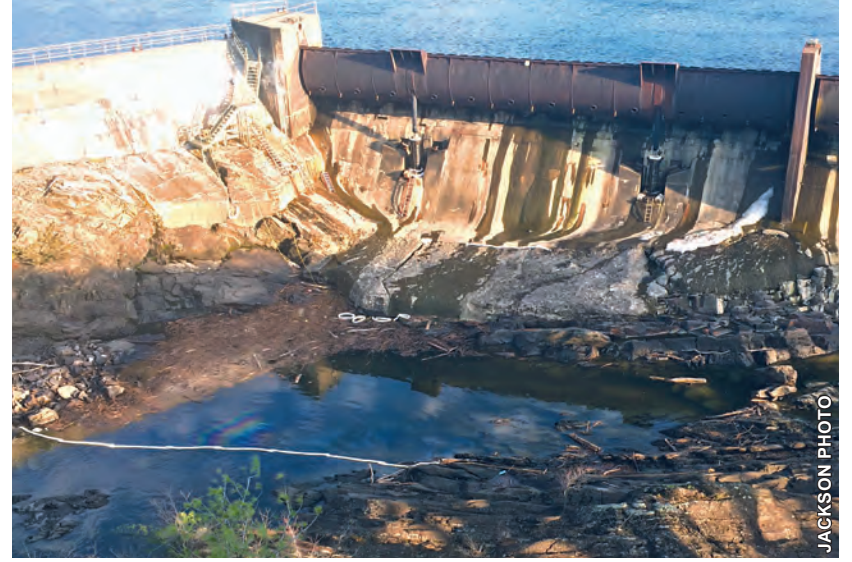
As of last weekend, an absorbent line was re-attached across the middle channel below Gate 4 to contain and help soak up a still-visible rainbow sheen of oil.
