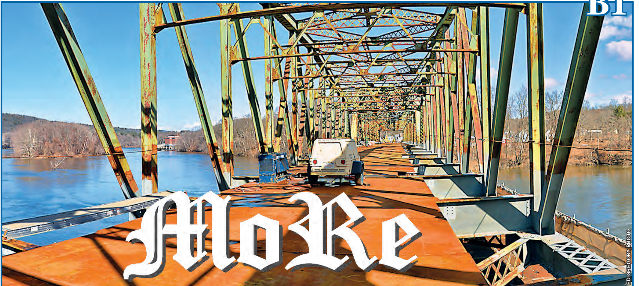
Above: Ed Gregory took this photo of the General Pierce bridge last week. “I’m near the west end of the bridge lookin’ east,” he writes. “The steel plates on the beams will serve as a temporary deck from which equipment will work to replace a series of removed beams. New beam segments will aid in supporting the sidewalk and railing along the south side of the bridge and the railing and curbing along the north side. The project is moving along nicely.” Thanks, Ed!
