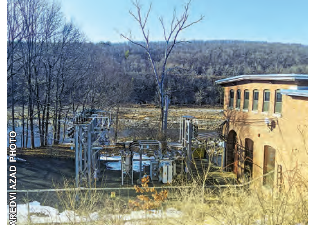
Turners Falls Station No. 1 would be updated to automate the flow through its turbines relative to that at the dam upstream.
