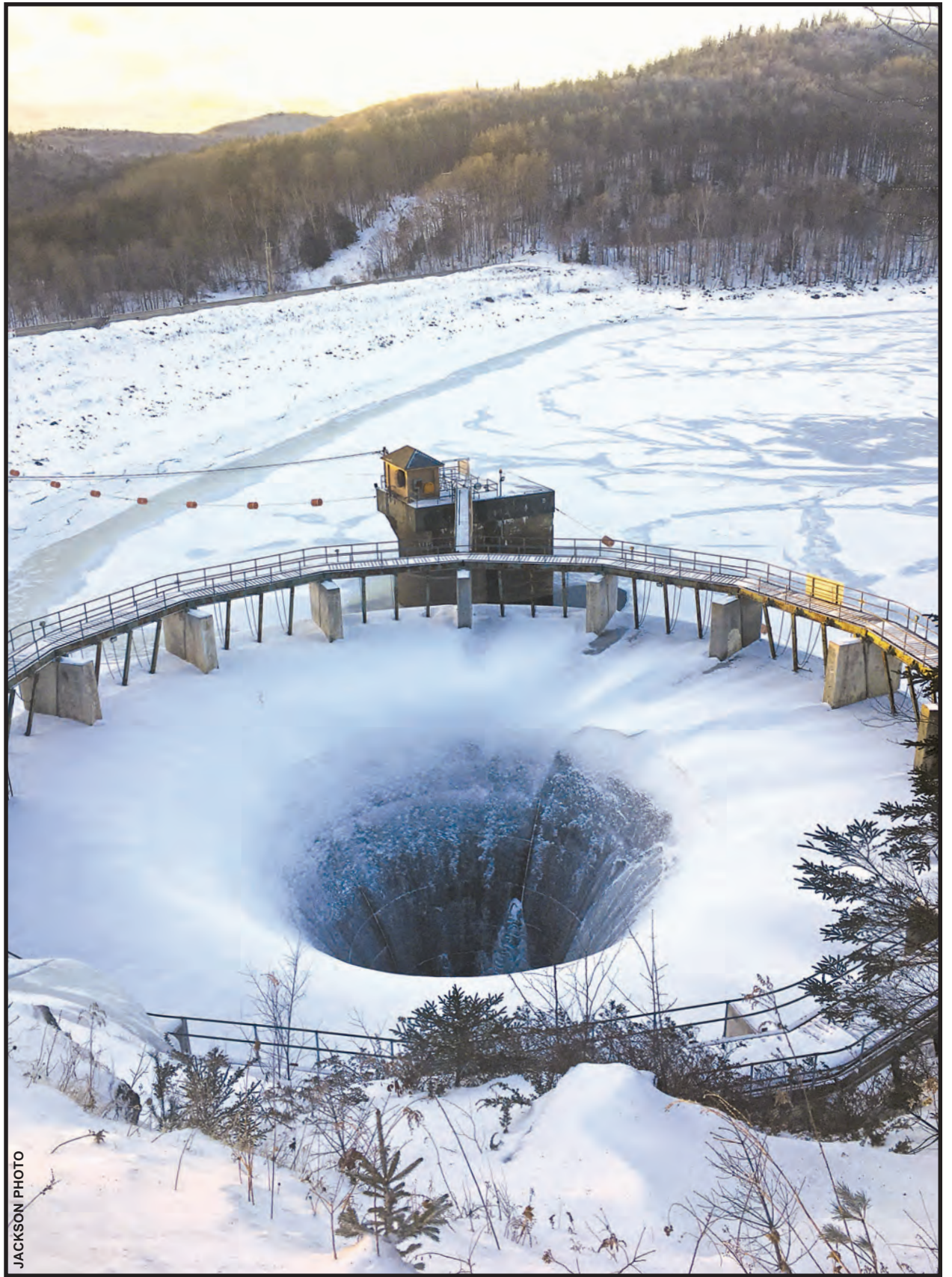
The "Glory Hole," a morning-glory spillway at the south end of the Harriman Reservoir, drains the Deerfield on warmer days.
