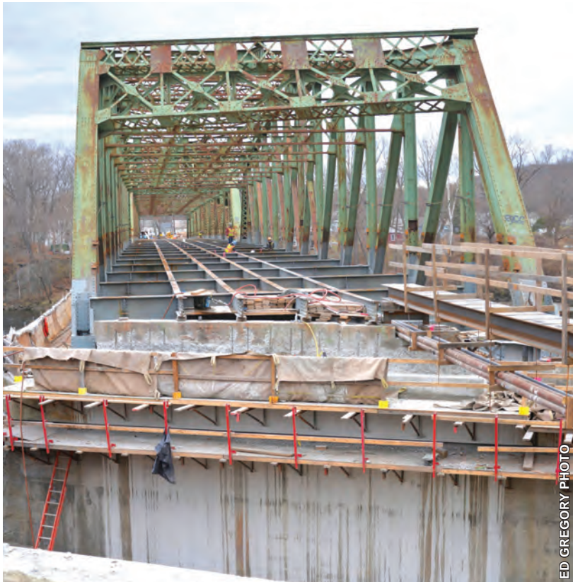
Ed Gregory took this photo of the work on the General Pierce Bridge last week from the Greenfield side. "It shows the westernmost pier section being demolished," Ed writes. "The old beams were of questionable integrity and have been removed. A new concrete pier section will support new beams that will connect the pier with the west abutment."
