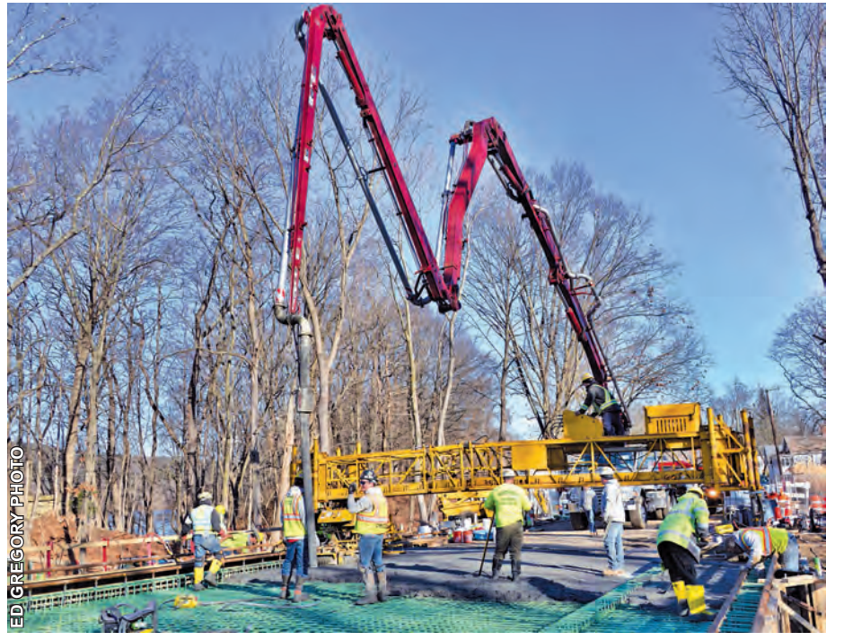
Photographer and historian Ed Gregory, our chief General Pierce Bridge correspondent, gave us another update Tuesday: "Deck paving machinery compacts, levels, and smoothes concrete fed to the deck via the segmented boom of the massive Baystate Concrete Pumping vehicle, which in turn is fed by the concrete mixing vehicle of the Chicopee Concrete Service Co.," he writes. "This line of trucks and machines will produce a new surface for the old bridge. The initial re-decking is on the east, or Montague City, end of the bridge. The first 60 feet will be completed today."
