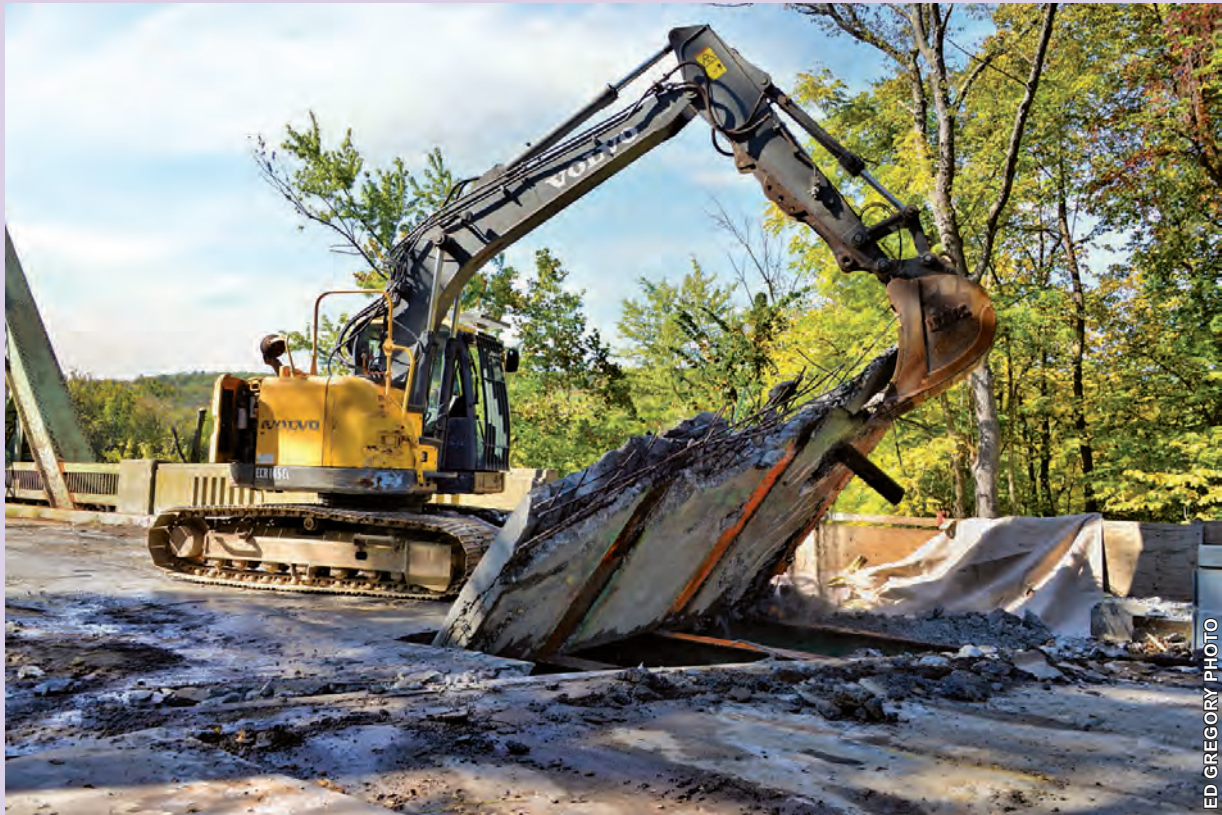
Deck work began in earnest on Tuesday on the General Pierce Bridge. The deck’s deterioration has been a subject of concern for several years, with a series of short-term fixes made before Northern Construction Services’s work started this spring.
