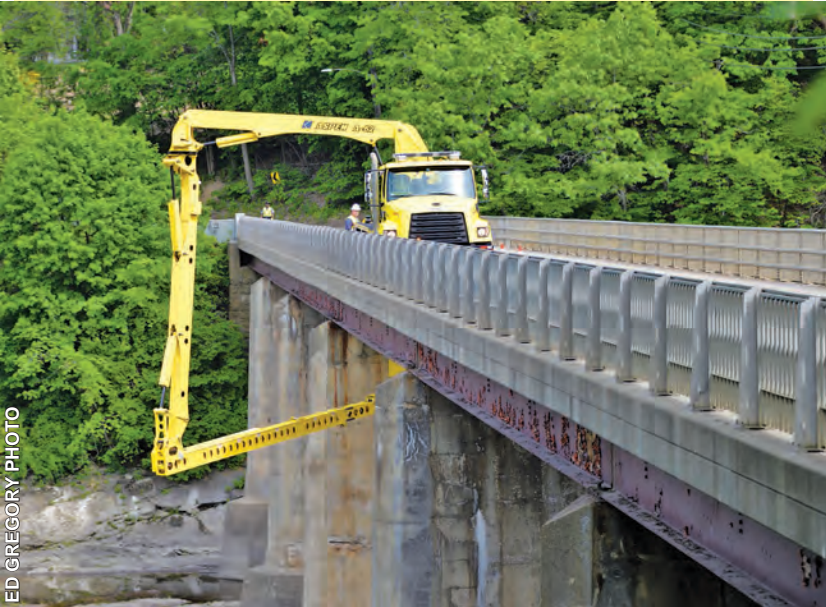
Above: Joe R. Parzych took this extra-close-up shot of Northern Construction Services' crew making progress on the General Pierce Bridge last month. The workers were preparing to work on scaffolding on the side of the steel-truss bridge. Below: Ed Gregory captured the "White" bridge undergoing an under-deck inspection on May 22. "After the upper or 'White' suspension bridge (1872) was destroyed by the flood of 1936, a replacement/temporary bridge was erected in its place in 1937... the bridge you cross today," Ed reminds us. Thanks to both photographers for their ongoing efforts to document the bridge work taking place around us this season, and sharing it with our readers!
