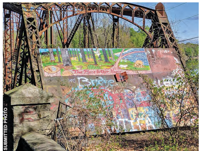
The Schell Bridge, slated for removal, and its newest mural.
