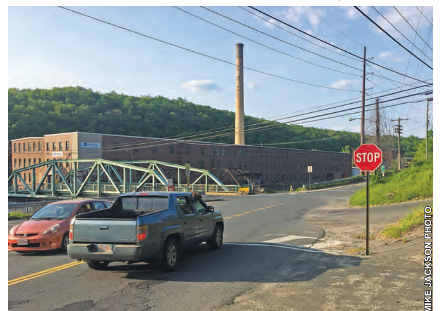
A recent Montague Reporter investigation confirmed that it is totally possible to blow right through the new stop signs at Canal and Fifth streets in Turners Falls if you don't know they're there. MassDOT installed the signs to deal with increased traffic at the intersection while the General Pierce Bridge is closed for repairs.
