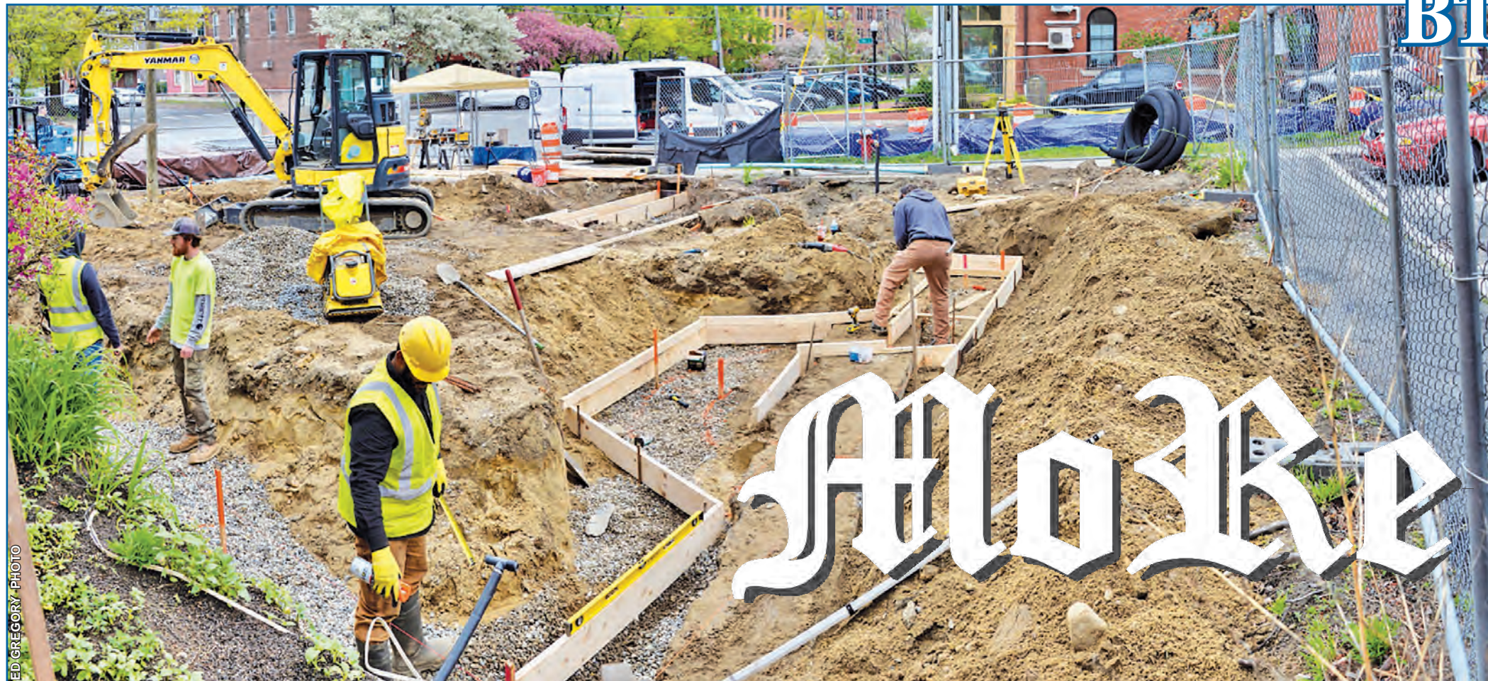
Above: Sciaba Construction of Waltham are deep into their rehabilitation of Spinner Park in downtown Turners Falls, building and placing concrete forms according to the plan designed by the Berkshire Design Group. Thanks to Ed Gregory for this photo!
