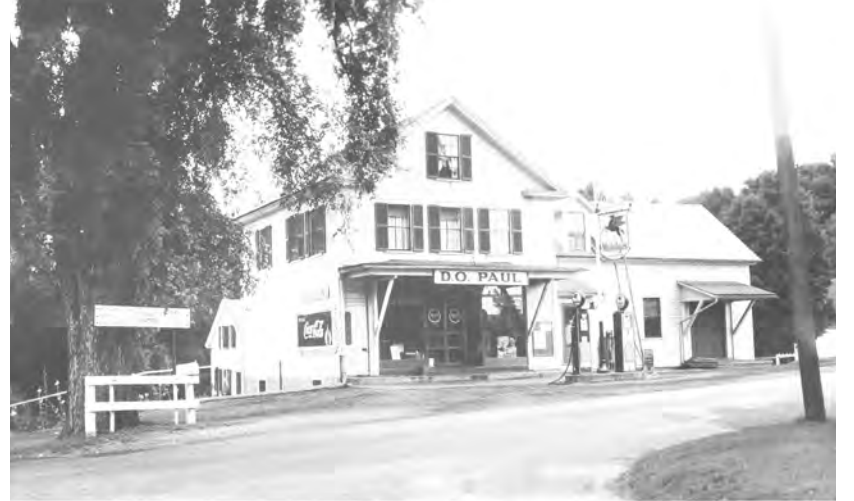
The D.O. Paul general store on Main Road, the present site of the Gill Tavern.
