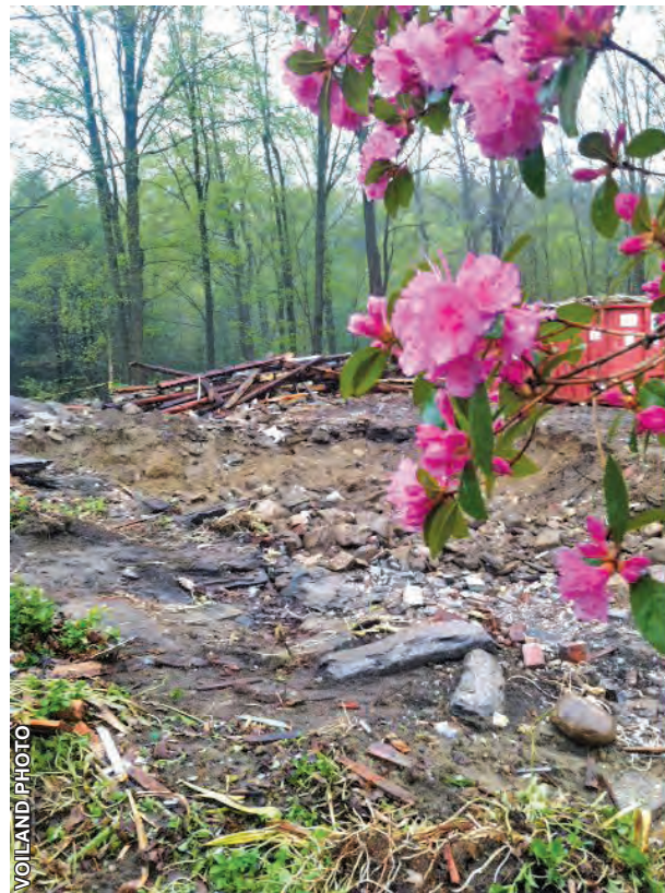
The cellar hole at the Montague Farm house, with a pile of its beams and a dumpster in the background.
