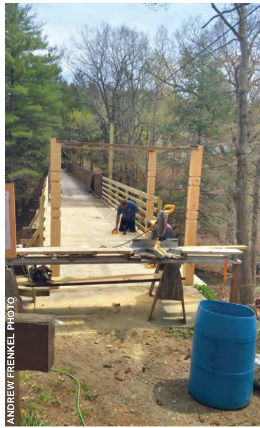
Work was underway Wednesday to rebuild the section of the Bridge of Names destroyed in an October windstorm.
