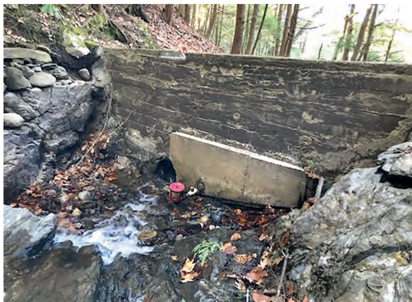
Top: Old Glory painted in a rock near the finish line of the annual great duck race. Bottom: Initially made of rock, the dam holding water was later reinforced with concrete. A pulley system was devised and the cement delivered bucket by bucket.
