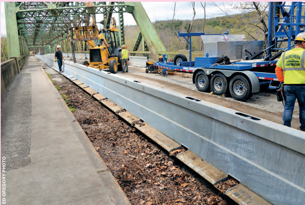
Work began this week on the General Pierce Bridge. The removal of the aluminum Jersey barriers is the first step.
