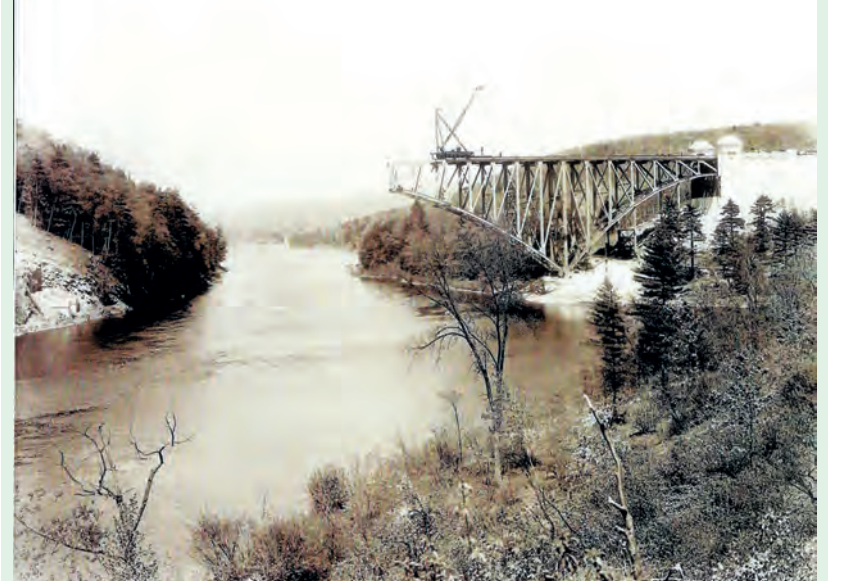
The French King Bridge was constructed in 1931 and 1932.
