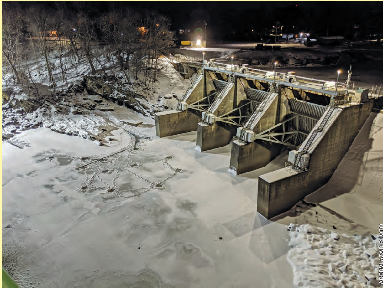
Above: Reader Aredvi Azad captured this image of the Turners Falls hydro dam's closed gates, illuminated at night.
