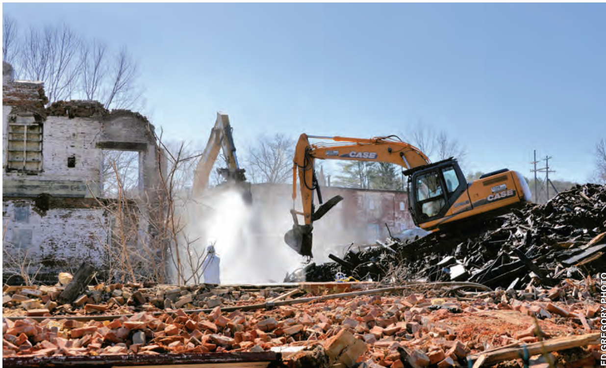
A pair of excavators move debris under a dust-quelling spray of water. The onetime Griswold Cotton Mill on Power Street in Turners Falls, widely known as the Railroad Salvage building, is being tidied up a bit this year by the federal Environmental Protection Agency. Environmental Restoration, LLC is handling the work. Thanks to Ed Gregory for the action shot!
