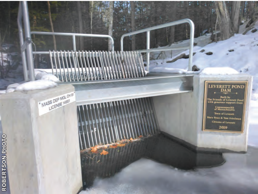
The pond's newly rebuilt dam makes a seasonal drawdown possible.
