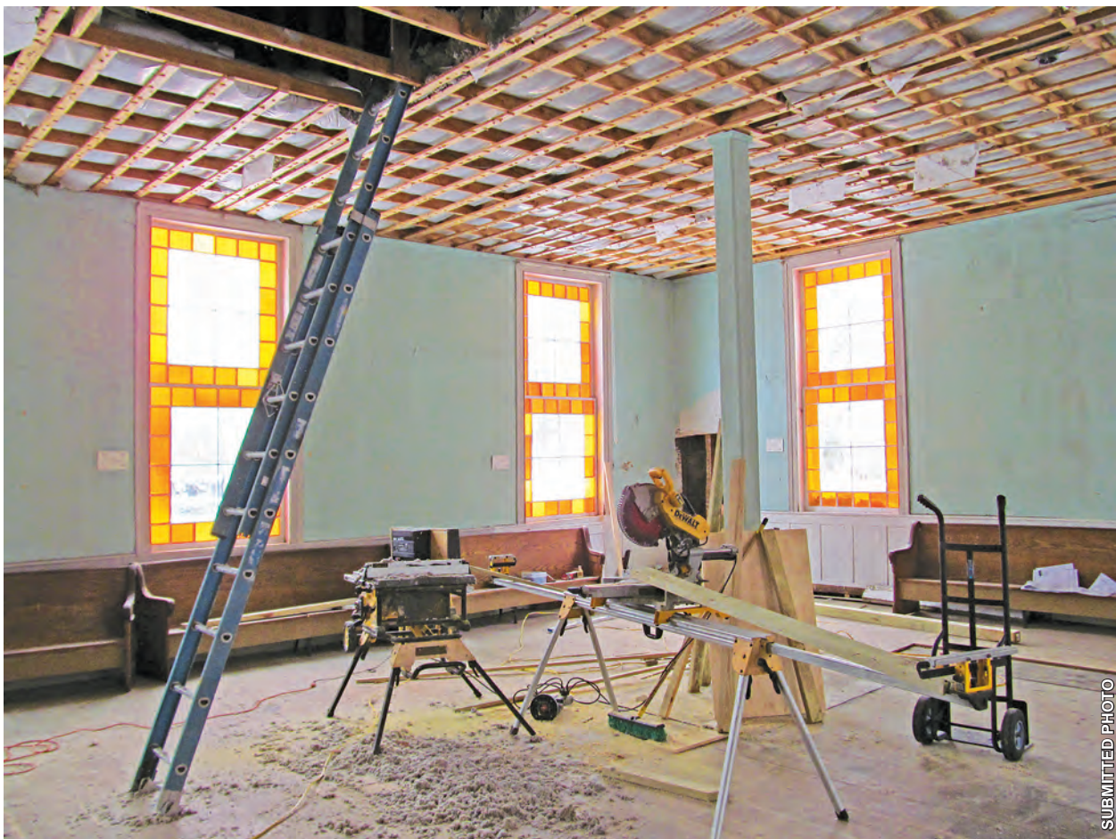
Restoration work gradually continues in the meetinghouse’s great room. The Friends aim to have the building ready for public reopening in time for Old Home Day next August.
