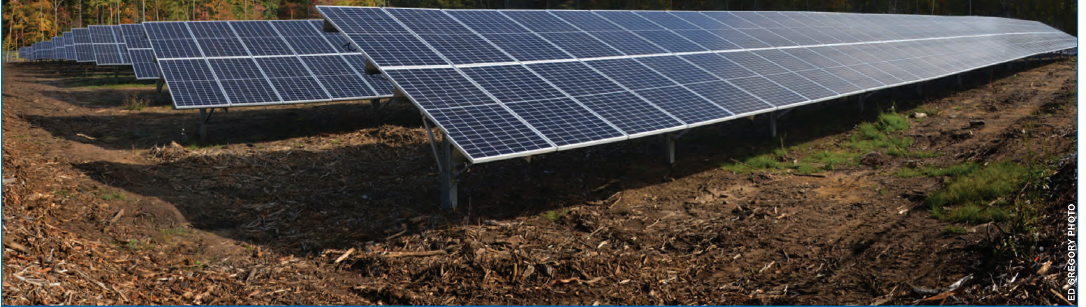
Above: Ed Gregory shared this photo of the solar array under construction on Millers Falls Road. The 2,710 photovoltaic modules take up 3.9 acres of the 4.2-acre lot. Thanks, Ed!
