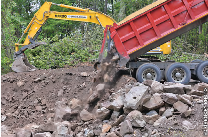
A truck dumps rocks down a Millers Falls Road embankment earlier this month. “When I was there on the 13th, the 186th truckload was dumped,” photographer Ed Gregory writes, adding that an engineer said the job was “about one-third complete.”
