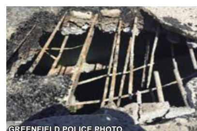
A 2015 hole in the bridge’s deck.
