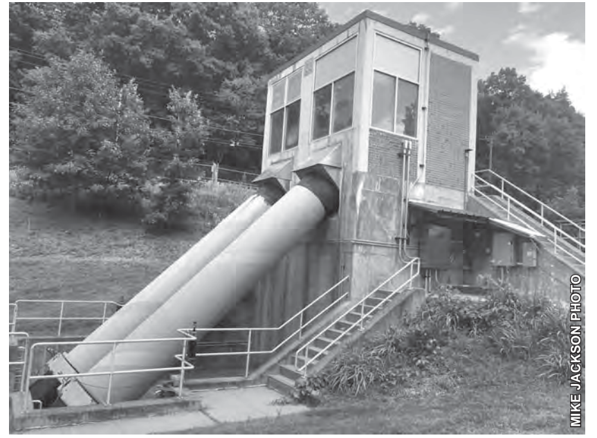
A pump station at the Montague water pollution control facility.
