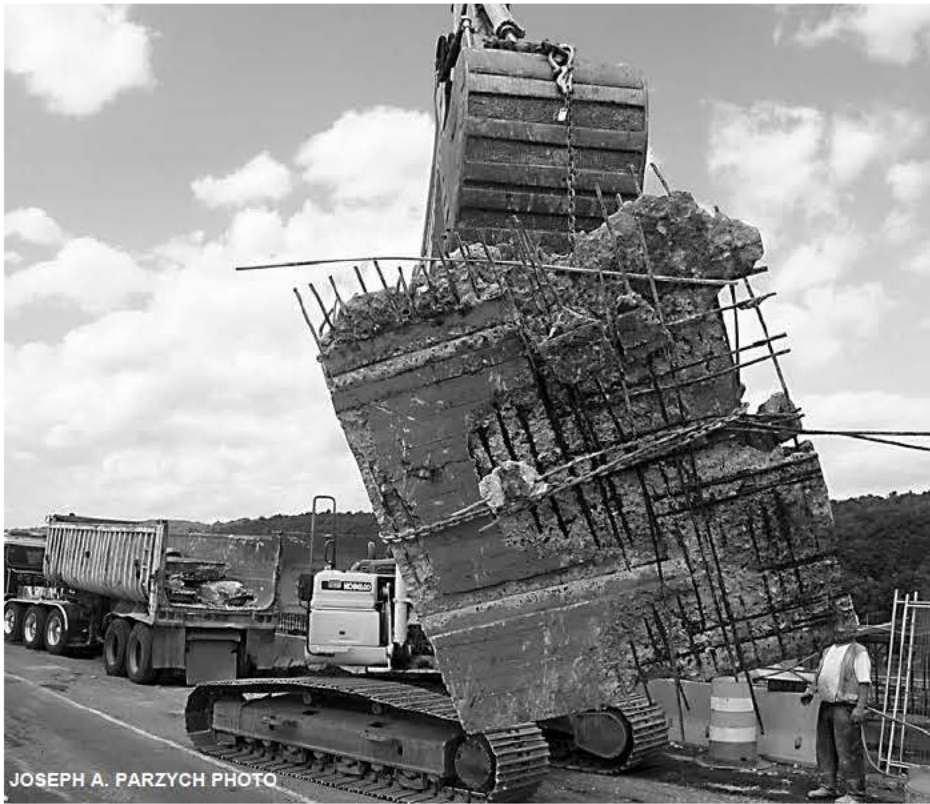
An SPS excavator carries a concrete slab from the bridge deck to a waiting 'bathtub' trailer with a barn door tailgate. The concrete is falling apart, and long overdue for replacement.
