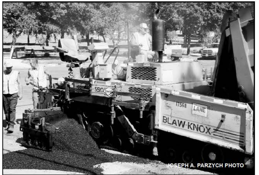
The Lane Construction crew lays down an inch and a half of fresh asphalt on Seventh Street and Avenue A on Wednesday
