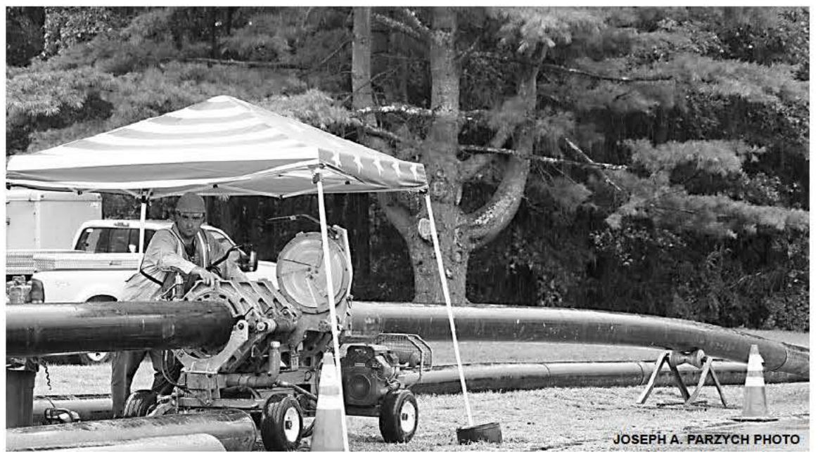
A worker at Northfield Mountain connects twelve-inch ABS plastic pipe with internal connectors in a pipe joining jig, sheltered from the rain on Ferry Road, by the pump house. A pipe of this diameter will be able to move a lot of slurry in a hurry from the clogged intake tunnel at the pumped hydro facility. The question is - where to put it, now that the EPA has halted FirstLight from discharging silt directly to the Connecticut River?
