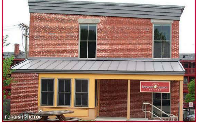
NEFC purchased this abandoned building for $1 from the town of Montague in 2006, spending half a million dollars to renovate it for workshop space.
