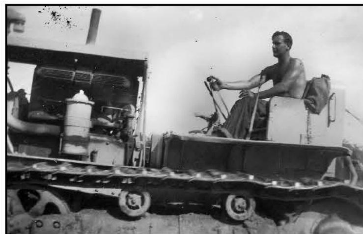
Charlie Yelton operating a dozer. a story by Sergeant Randy Hanes Mud Hill in Belgium
