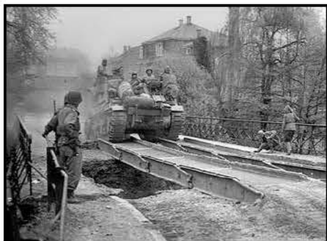
First Bridge Constructed by C. Co. - 300th Engineer Combat Battalion A temporary treadway across the Douve River, Pont L'Abbe, (4 miles SW of Ste-Mere Eglise) Normandy, France, June 18th, 1944
