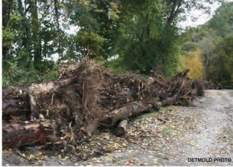
Stockpiled woody debris waits to be installed to stabilize the bank of the Connecticut River at the Lower Split River Farm site in Gill.
