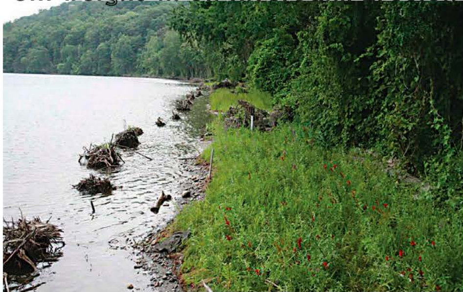
Woody debris is anchored by the bank of the Connecticut to prevent erosion in Gill.
