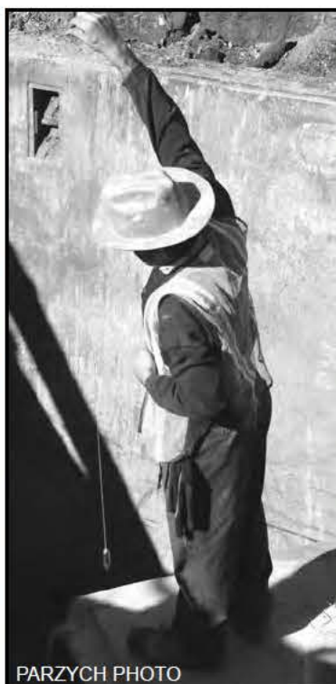
Lining up the pipe on Ave A
