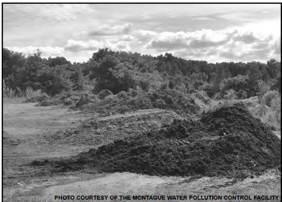
Mounds of debris removed from a 150-foot sewer pipe that had been installed years ago on a positive incline, from the Greenfield Road combined sewer overflow structure to the headworks of the treatment plant. The pipe was more than half filled with sediment, and had not been cleaned out in nearly three decades. WPCF superintendent Bob Trombley said the flow to the headworks is now much improved.
